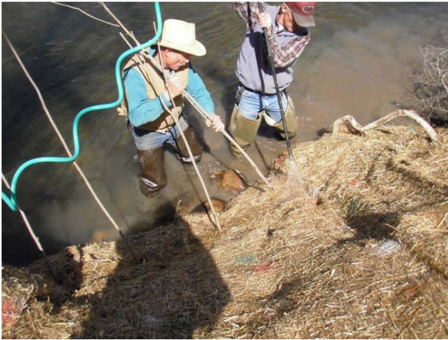
Waterjet Stinger in operation during stream bank re-vegetation. Photo supplied by Carrie Rogaczewski, SCCD
